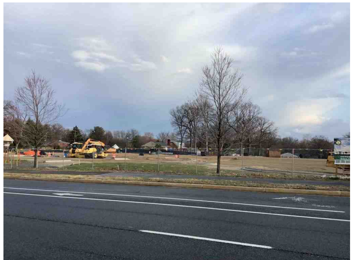
Church being built east of the subject
