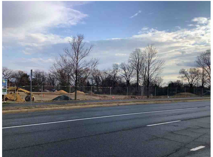
Church being built east of the subject
